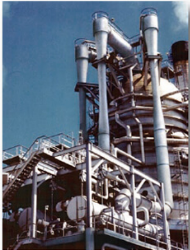
Vacuum Distillation Column
